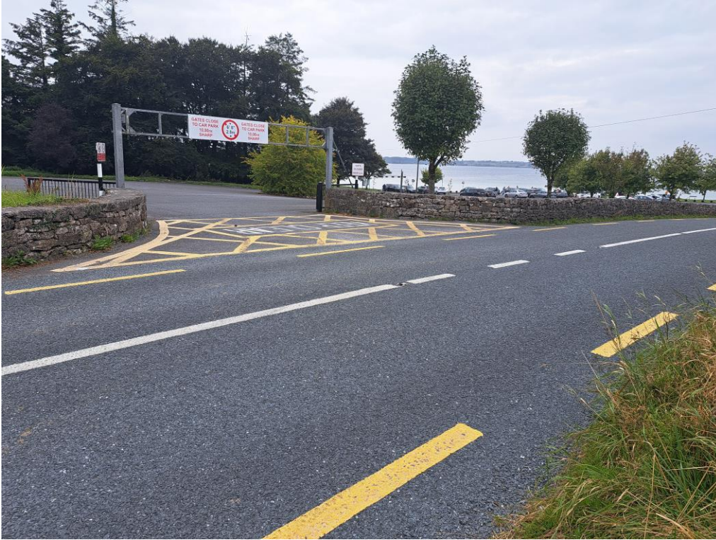
Plate 3 Existing southern access (furthest from Loughrea)
