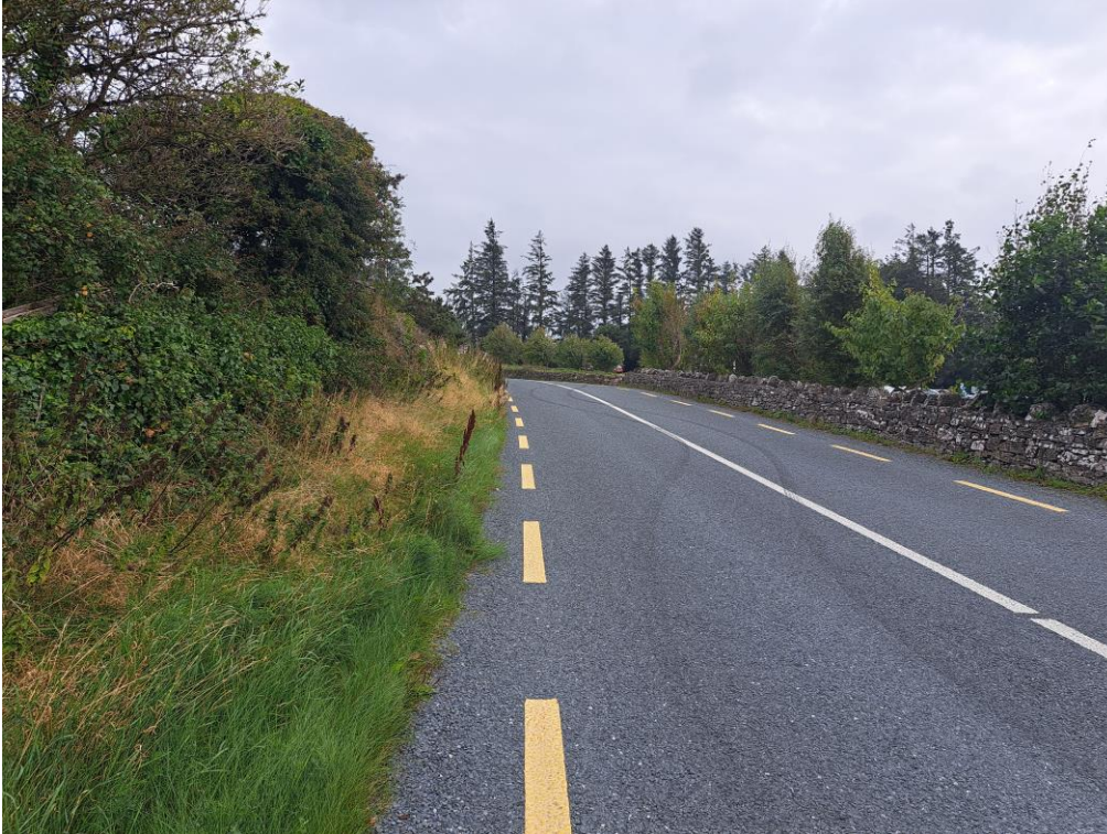
Plate 8 Existing northern access – Looking south along R351
