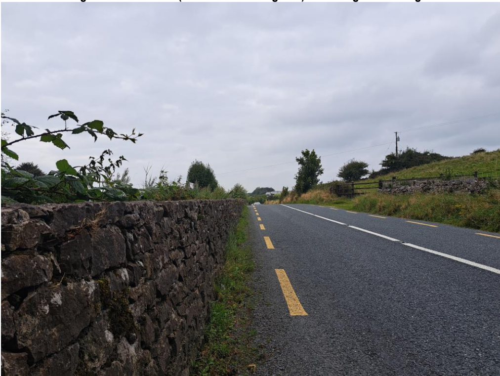
Plate 4 Existing southern access (furthest from Loughrea) – Looking north along R351 with access on left
